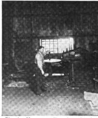
Circular Shear rounding plates for the saw factory
