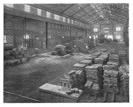
Cogging Mill with ingots ready to reheat
